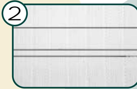
3) Chalk all three lines. The upper two are the cut lines. Cut vertically on each side of the web to create a pocket 6" (150mm) wide. Cut out EPS pocket. The lower horizontal cut should be on an angle (45 degrees) to facilitate the concrete placement. Key hole saw, reciprocating saw or hot knife are best for this task. (see 3)
