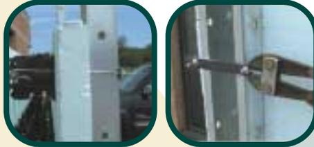
12. When removing cross braces, unscrew the nuts when the connection wires are still required. When the connection wires are no longer required, they can simply be cut. Use the same cutters to remove as much of the wire as possible in the finished wall.
