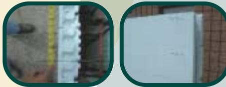
4. Measure for the width of the scaffolding and place the second set of connection wires on either side of the channel or scaffold.
