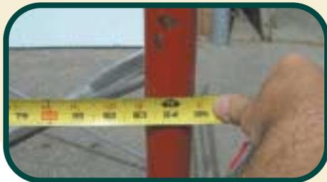
1. The NUDURA Tall Wall Adaptor Kit can be used with any conventional scaffolding. Measure the width of the scaffolding being used and transfer.
