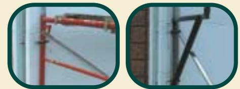
9. We recommend that all of the cross braces are applied to the channels and at least the top and bottom cross brace for the scaffolding. When the channel is securely attached it may be used in the typical fashion.
