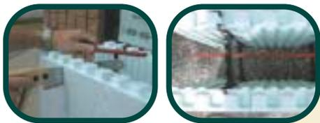
2. Cut two slits in the form with hand saw. Place cuts on either side of the channel or scaffold.
