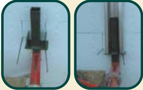
10. Insert the channel to the scaffold adaptor into the end of the scaffold frame and secure using a pin or a nut and bolt.
