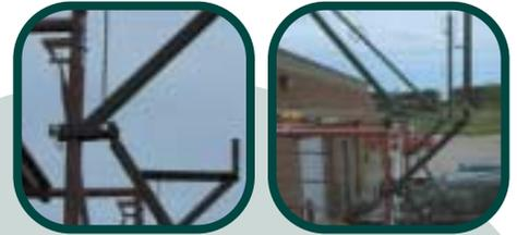
13. Insert the turnbuckle adaptors into the free end of the scaffold frame. Use the spring pin to secure the bottom of the frame and insert a pin or bolt through the aligning holes of the frame. Once in place, the guardrail posts and turnbuckles can be installed. The pad of the turnbuckle attached to the channel slides into the adaptor and is secured by a pin and clip.
